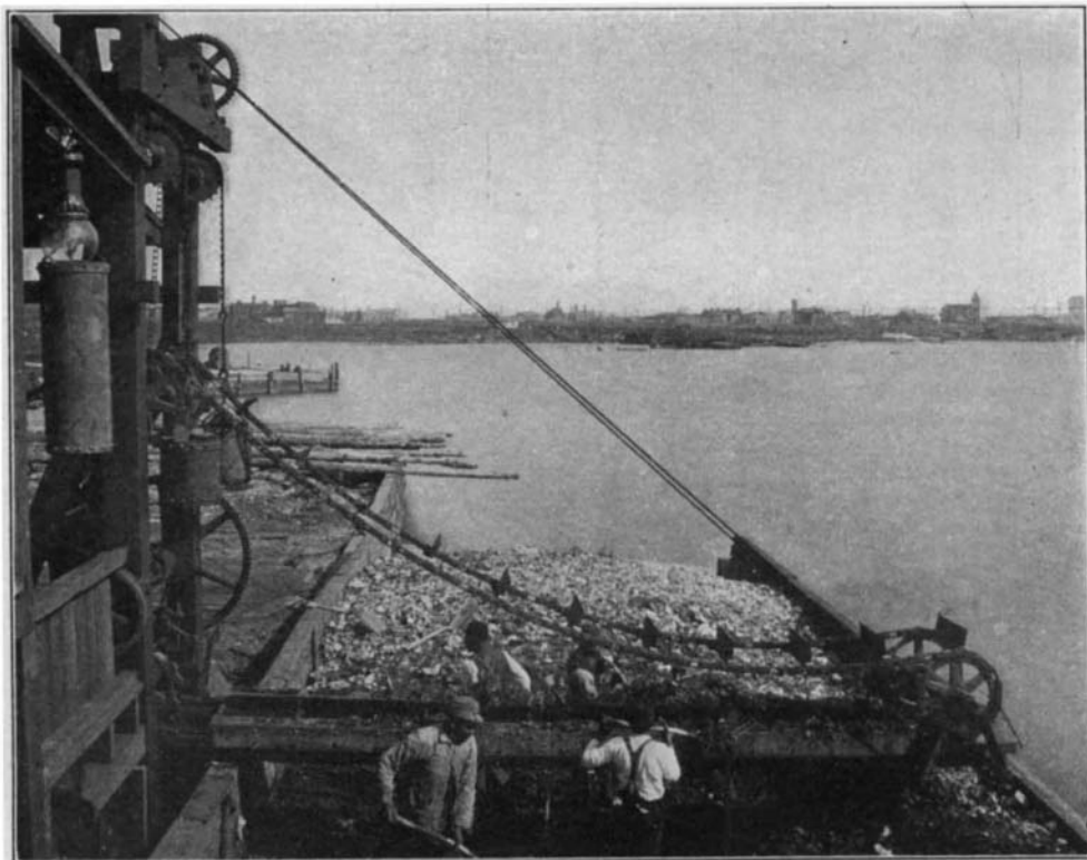
Automatic Conveyor for Unloading Garbage.
