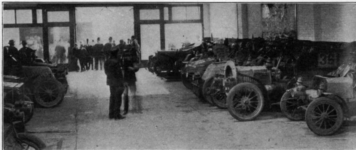
The Automobiles Stored in the Official Garage at Pittsburg.
