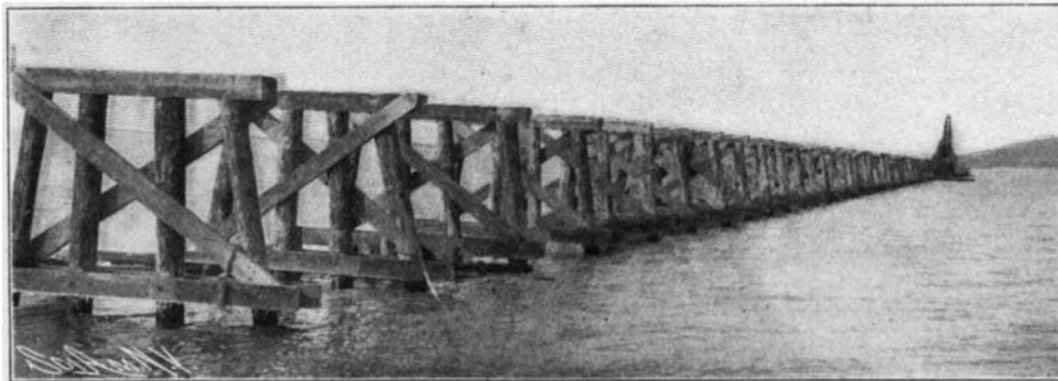
Framework of Trestles Which Collapsed.
