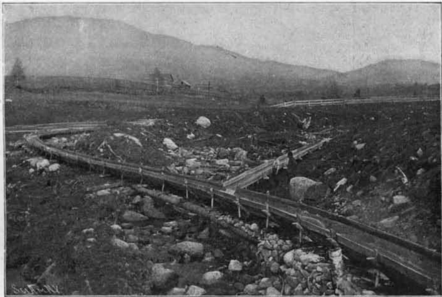
A Lumber Slide, Showing a Feeder.
