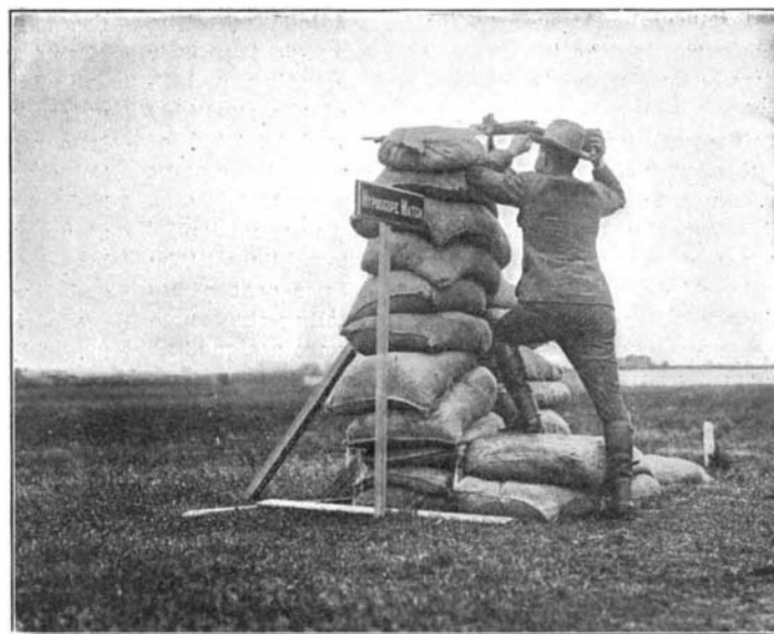
Aiming with the Hyposcope Over Breastworks.
