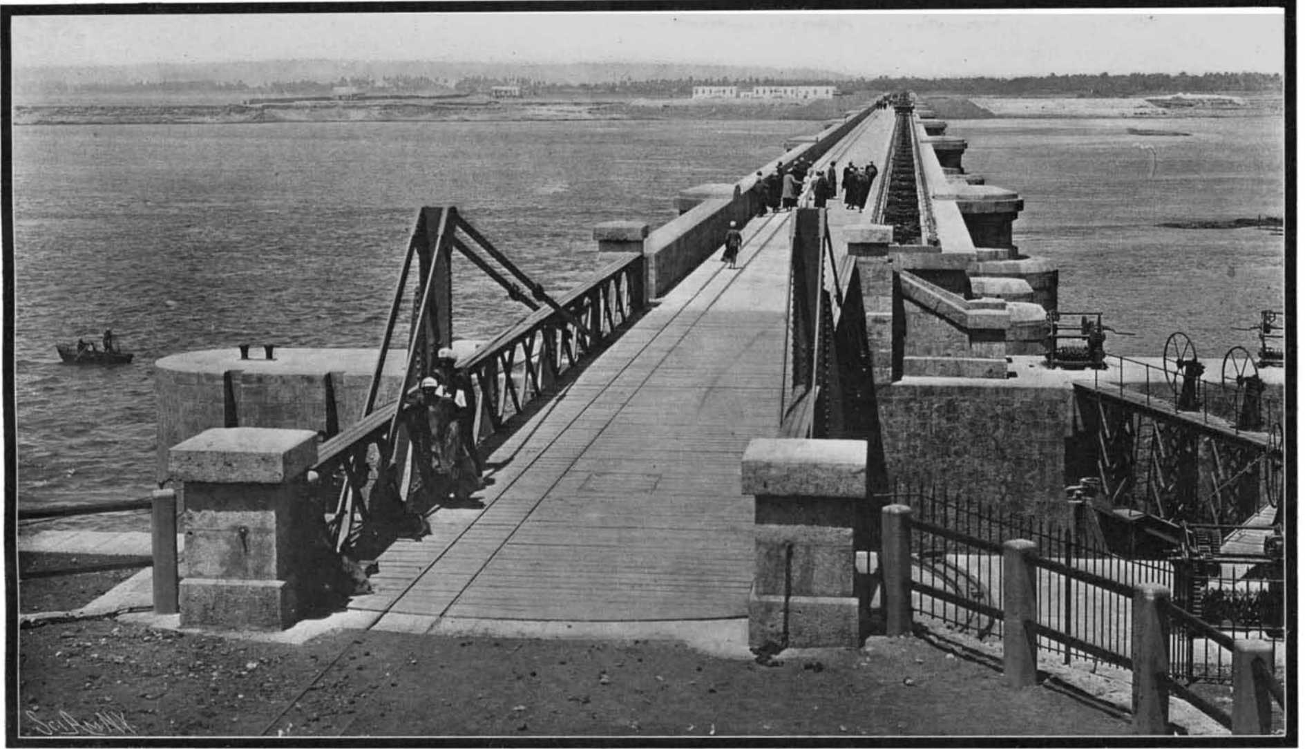
View Looking East Along the Roadway, showing Track for Sluice Regulating Gear.
