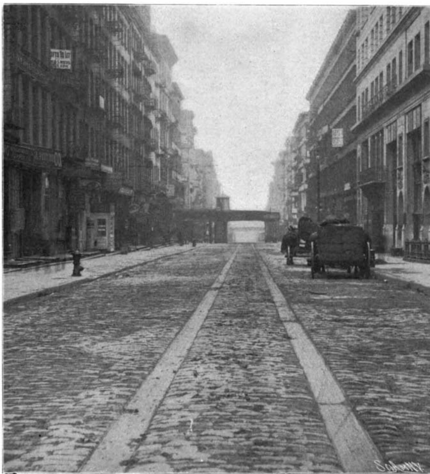
APPEARANCE OF STEEL ROADWAY IN MURRAY STREET, NEW YORK.
