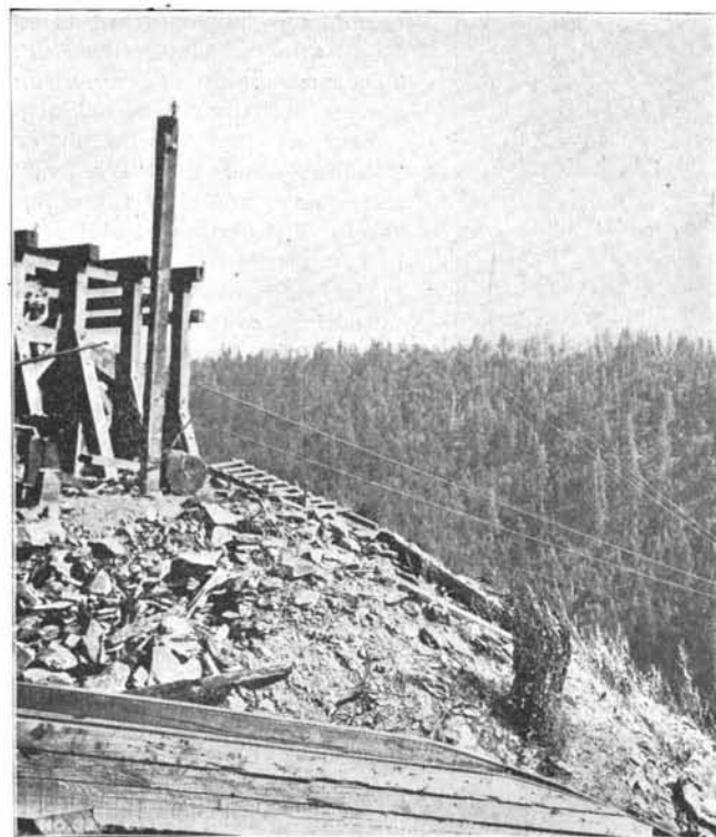
Head House and Cables.
