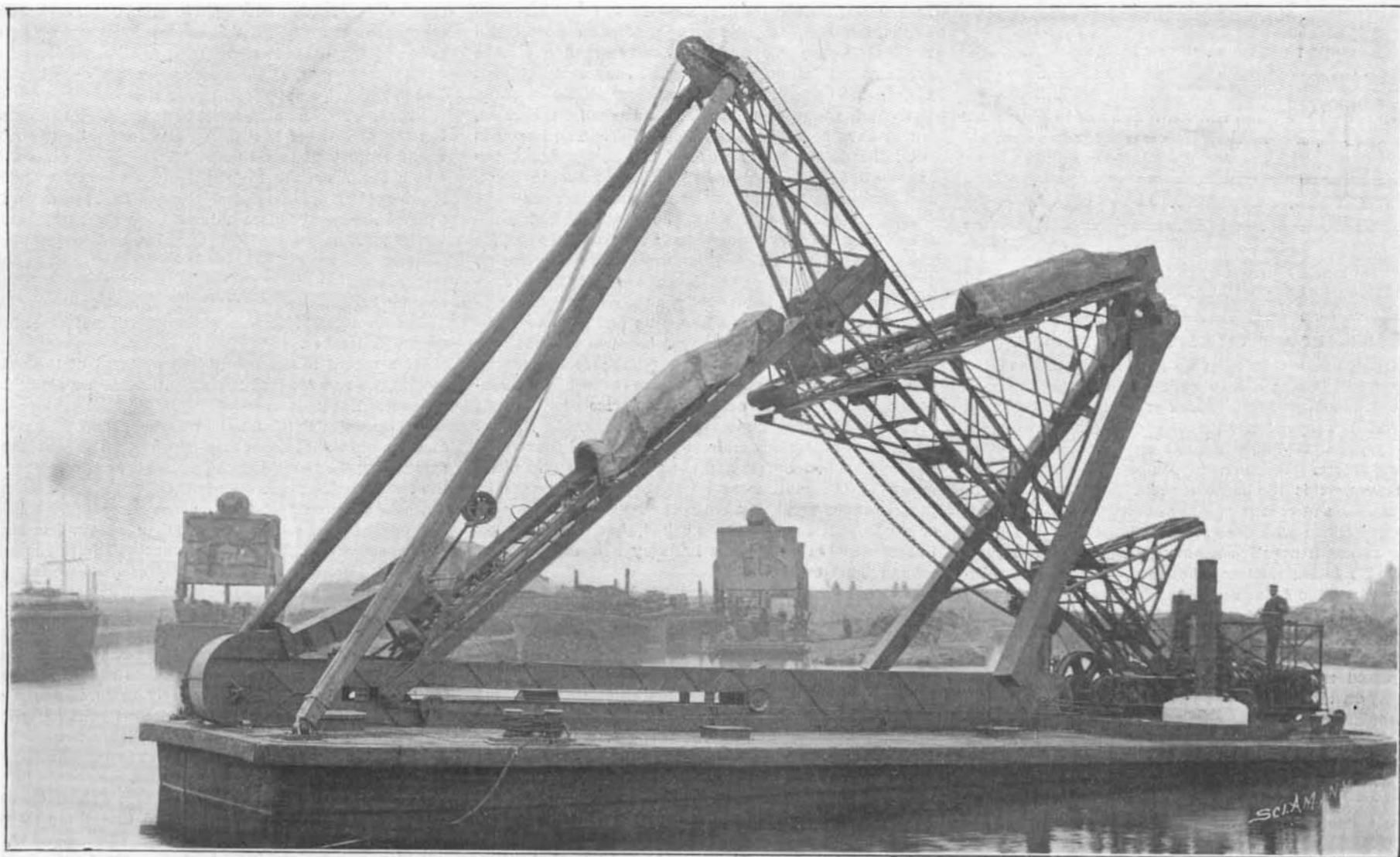
"Grasshopper" Elevator in Housed Condition.
