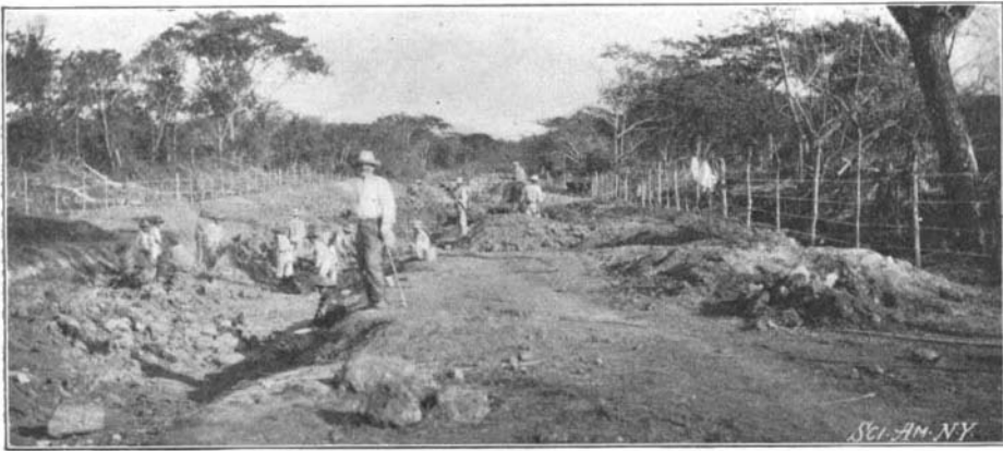
Right-of-Way Cleared and Grading Under Way.
