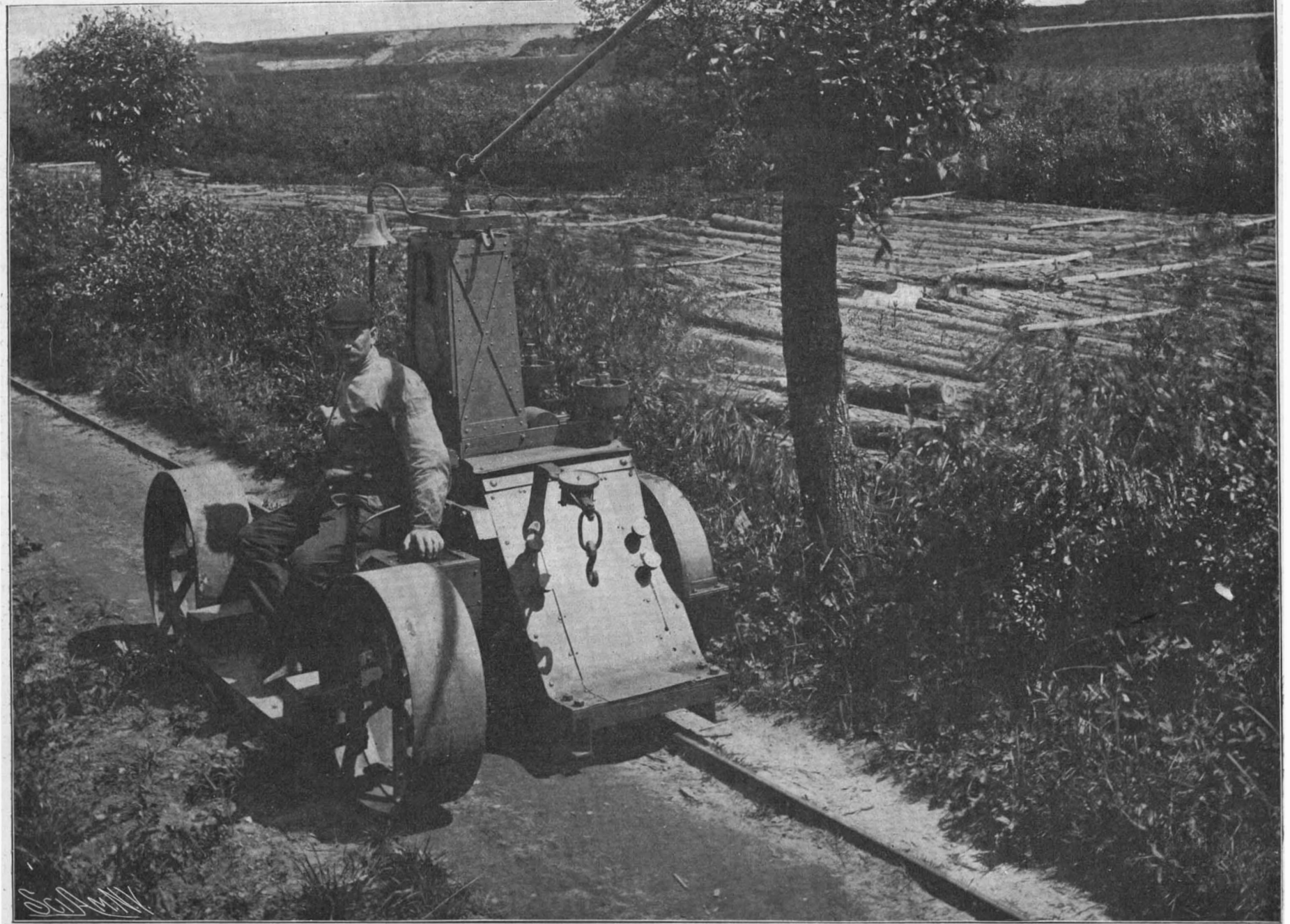
TOWING BARGES BY ELECTRIC LOCOMOTIVES ON A GERMAN CANAL.—[See page 483.]
