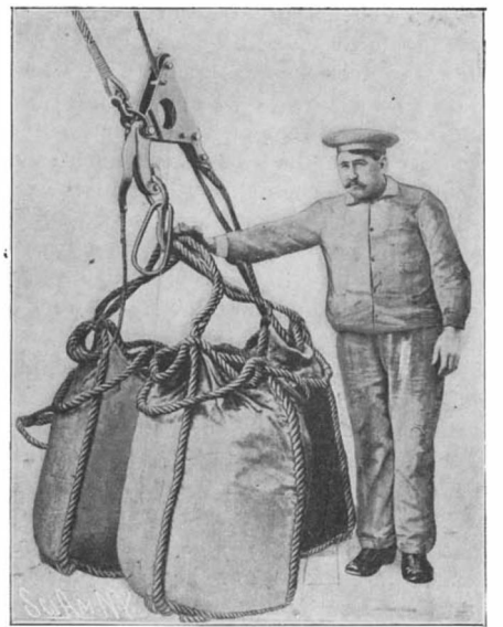
Elevating Truck Loading Bags on the Deck Ready for Hoisting to Masthead.
