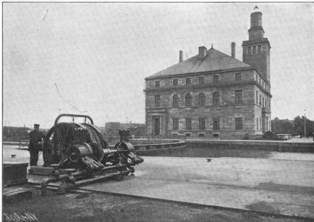
GATE-OPERATING MECHANISM AT SAULT STE. MARIE.
