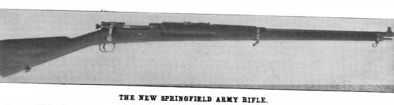
Muzzle velocity, 2,300 feet per second. Weight of bullet, 220 grains. Weight of charge, 43.3 grains. Weight of gun including bayonet and scabbard, 9.47 pounds.
