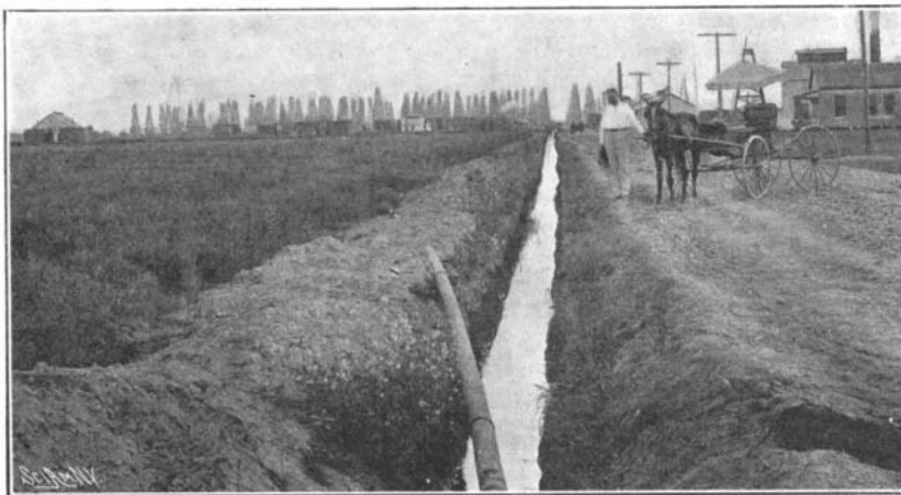
A Typical Pipe Line, and an Open Ditch for Conveying Oil to the Earthen Reservoir
