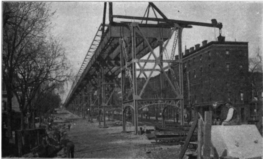
Manhattan Valley Viaduct, Showing Skewbacks for Arch.
