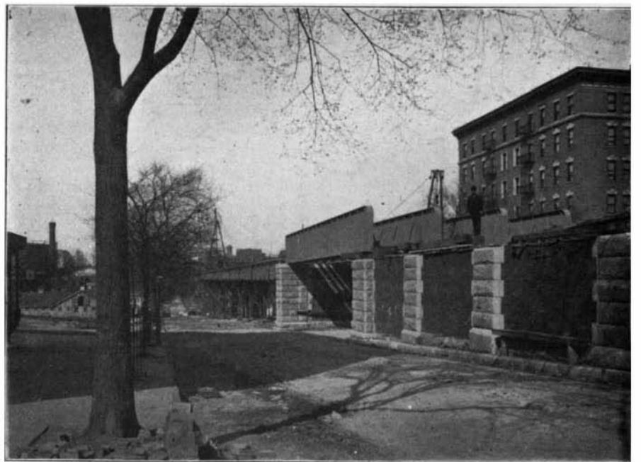
Masonry of North Approach to Manhattan Valley Viaduct.
