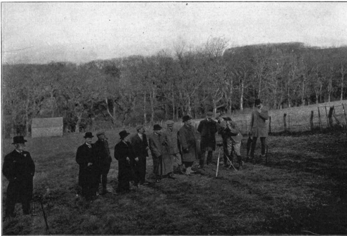
DETECTING THE EARTH CURRENTS SENT OUT BY THE TRANSMITTER.
