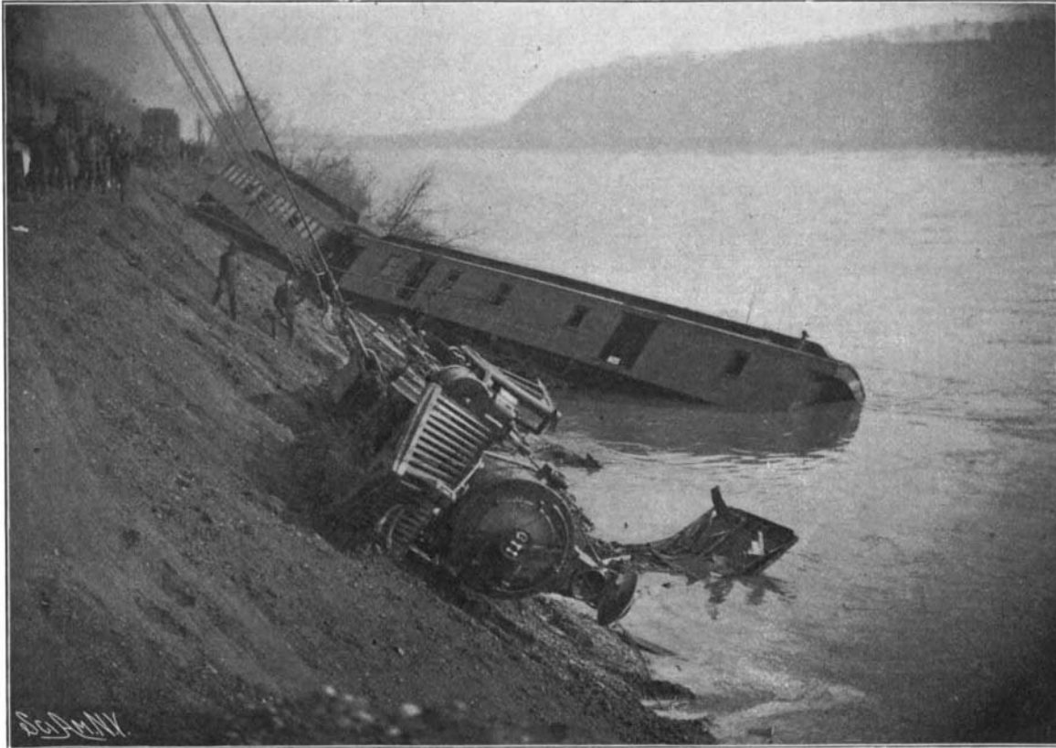
RAILROAD WRECK NEAR PITTSBURG. DOUBLE CRANE HAULING A 50-TON LOCOMOTIVE FROM THE RIVER.
