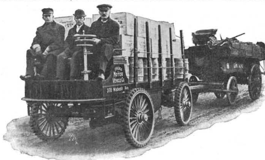
Auto-Truck, 2 to 4 Tons Capacity (Furnished with Enclosed Vestibule Front)
