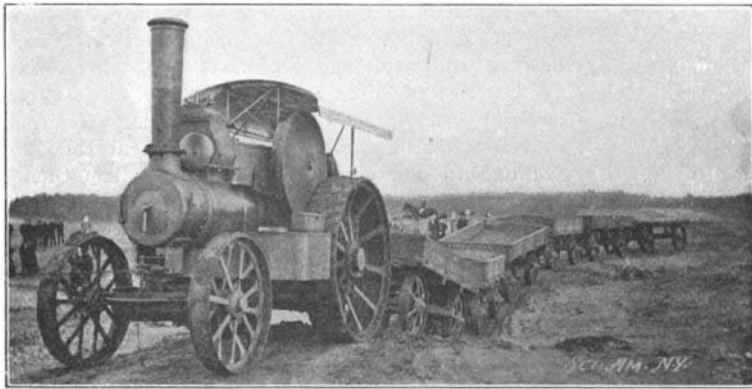
Hauling a Train Over a Gully.
