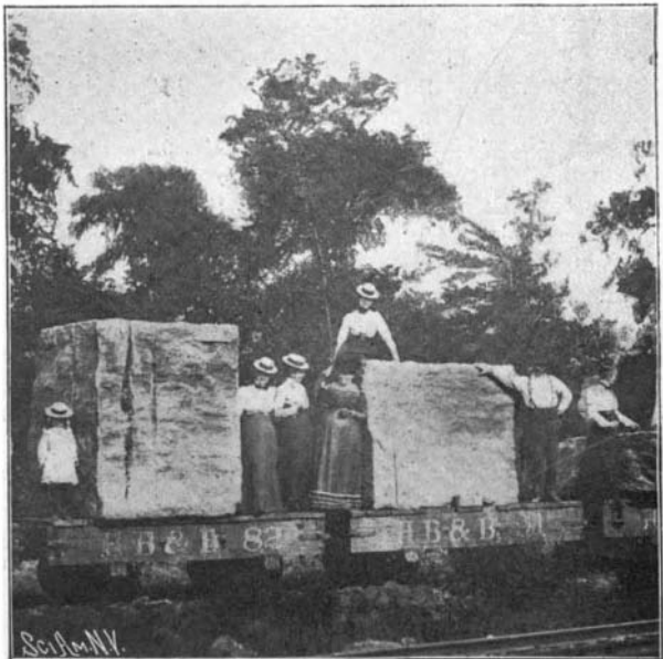
Trainload of Large Capping Stone, Ready for Shipment to the Breakwater.
