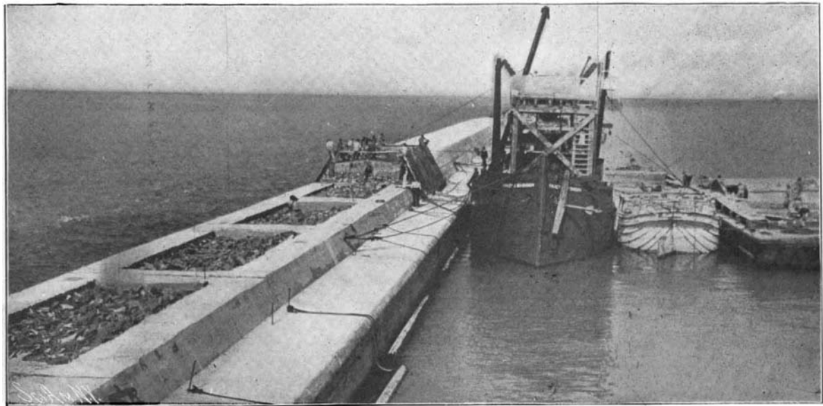
Building Concrete Structure Above the Timber-crib Foundation.
