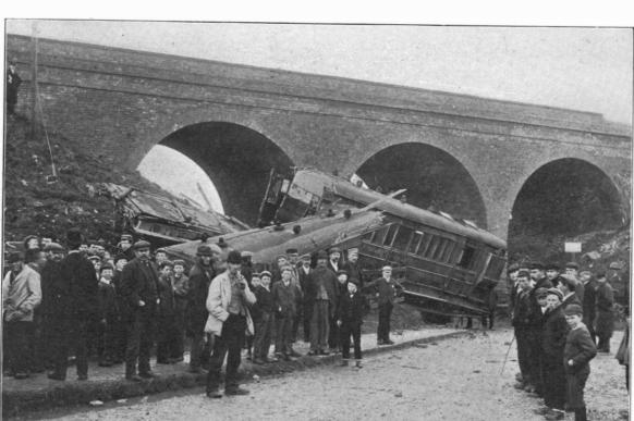
THE WRECK AT LITTLE BYTHAM. THE TRAIN LEFT THE VIADUCT BECAUSE OF THE SPREADING OF THE RAILS.
