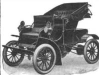
1903 Model now ready, with many new and desirable features. Wood Wheels, 34-in. Double Tube Tires, Longer Wheel Base, More Powerful Air-Cooled Engine, Wider and More Comfortable Folding Front Seat easily carrying two adults. Price \$1,200.
