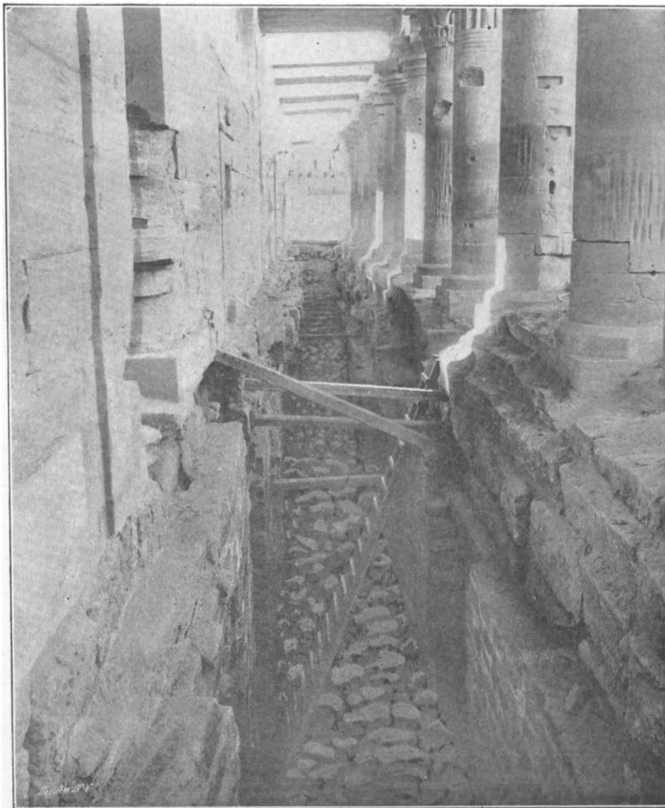
COLONNADE LOOKING SOUTH. READY FOR THE LAST LENGTH OF MASONRY. THE TRENCH IS PARTLY FILLED IN AT THE FARTHER END.
