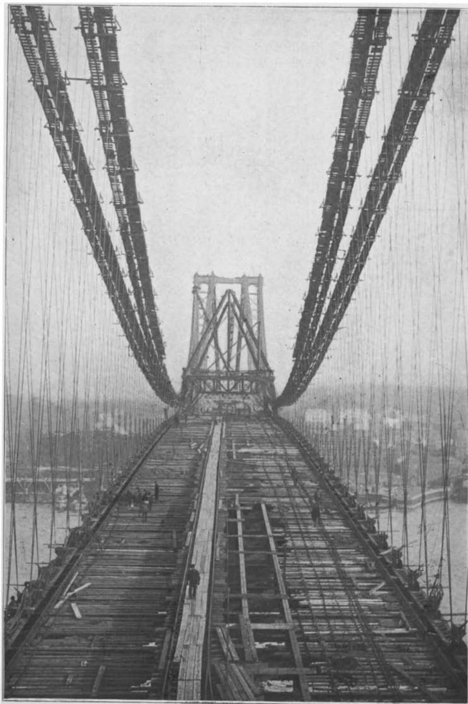
View Looking Along Axis of Bridge, Showing the Floor Between Cables Erected. Cantilever Extensions of the Floorbeams, Extending 20 Feet Beyond the Cables, will be Bolted on, Making a Total Width of Floor of 120 Feet.
