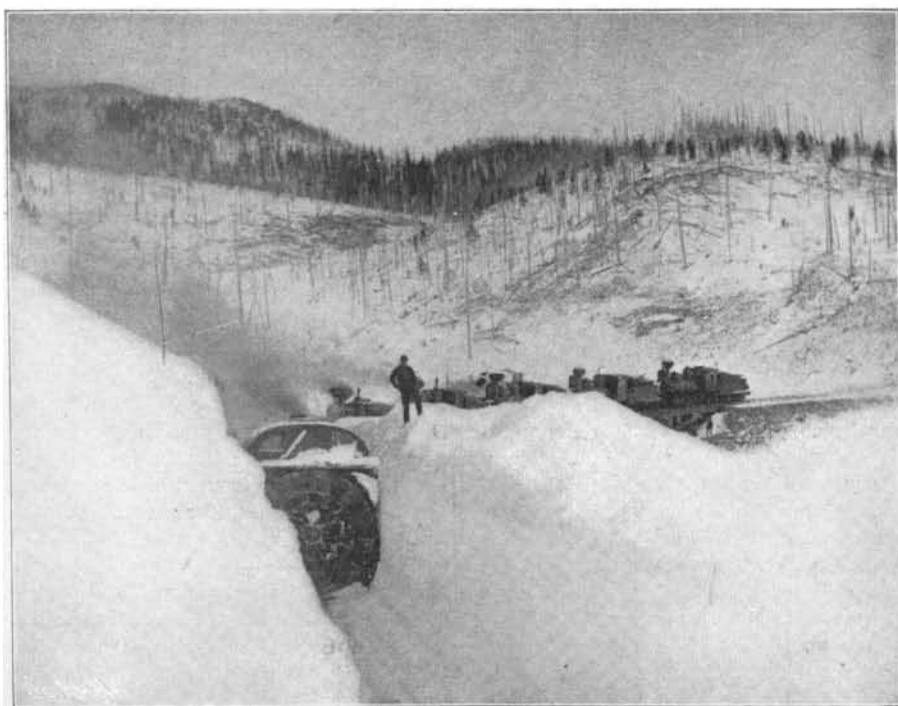
A ROTARY PLOW IN TWENTY FEET OF SNOW.
