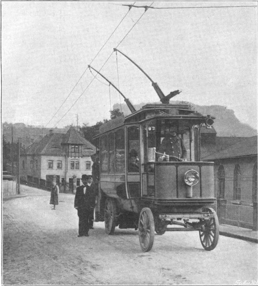
Electrical Trolley Omnibus and Power House.
