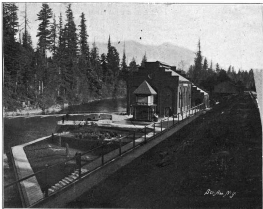
The Headworks Above the Falls, Showing Intake, Transformer House, etc.
