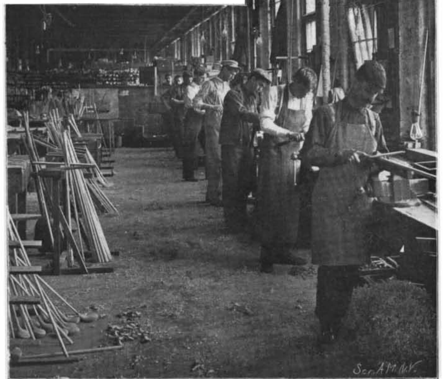
Finishing the Shafts with File and Sandpaper.
