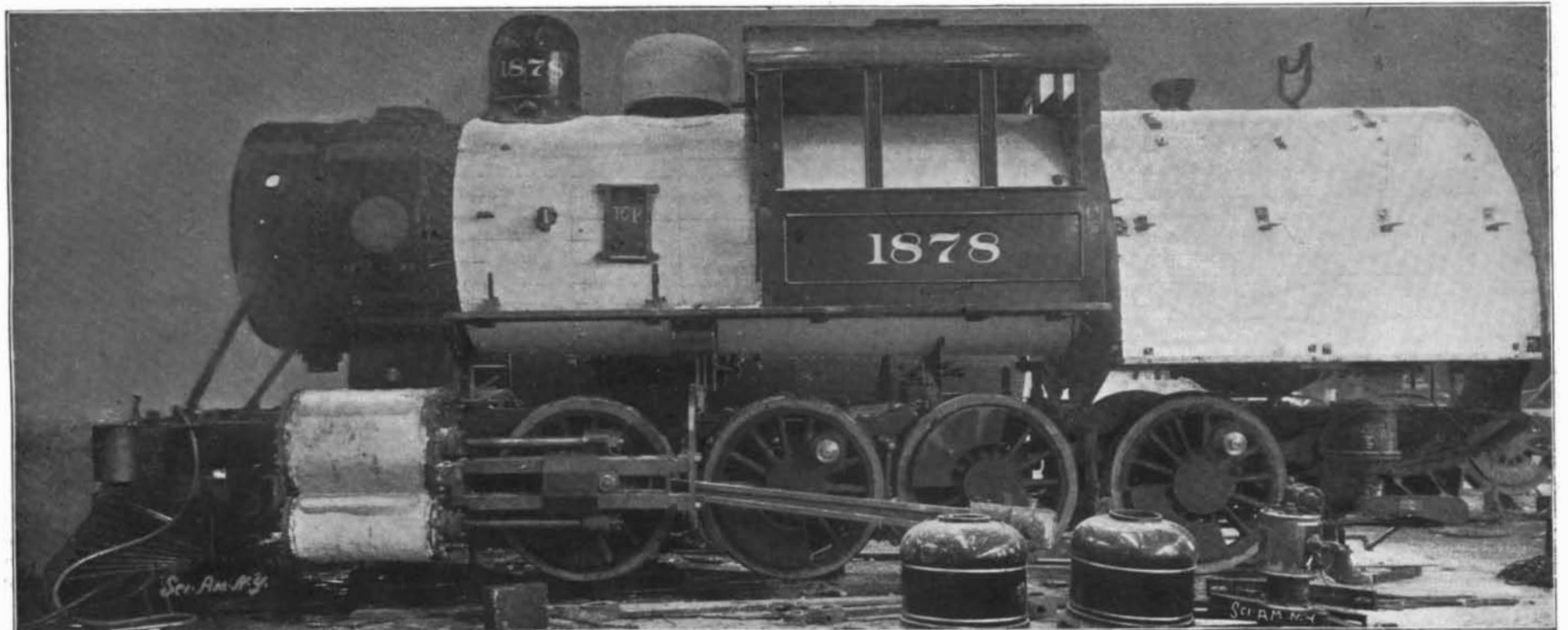
Fourth Stage of Locomotive Erection: the Boiler and Cylinders Lagged with Magnesia.
