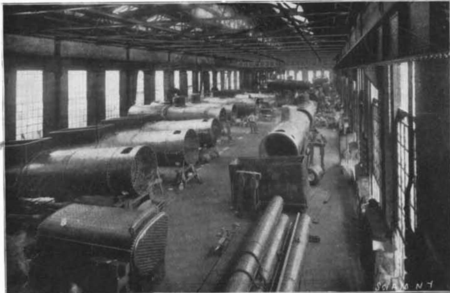
The Boiler Shop.
