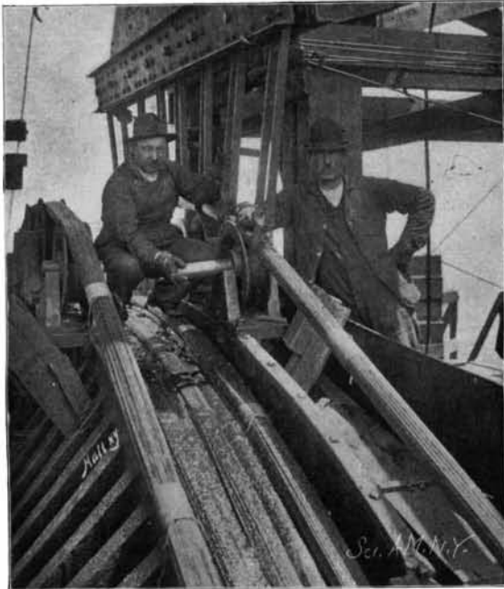
Binding Wire Strands Into Cables.
