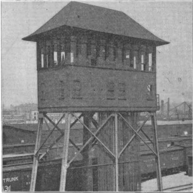
Fig. 5.—Signal Cabin at the Grand Central Station, Chicago.
