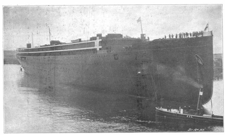
Length, 70614 feet; breadth, 72 feet; depth, 44 feet 2 inches; displacement, 26,000 tons; contract horse power, 40,000; estimated speed, 2314 knots,
