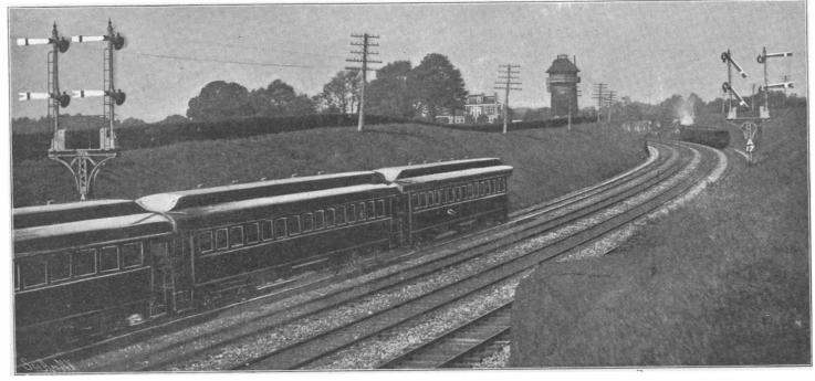
Fig. 4.—Westinghouse Electro-Pneumatic Semaphore Block Signals on the Pennsylvania Railroad. BLOCK AND INTERLOCKING SIGNALS.
