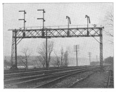
Fig. 2.—Grafton Three-position Automatic Block Signals on the Pittsburg, Fort Wayne and Chicago Railroad.
