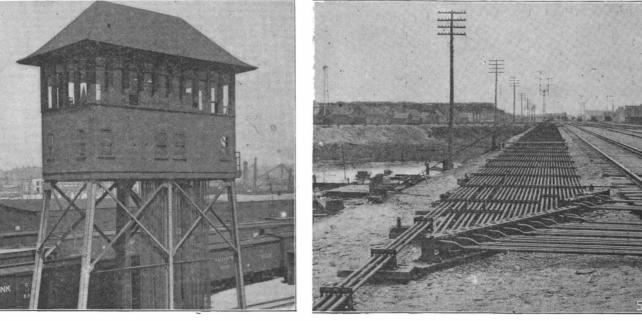
Fig. 6.—Connections from Cabin to Switches and Signals.
