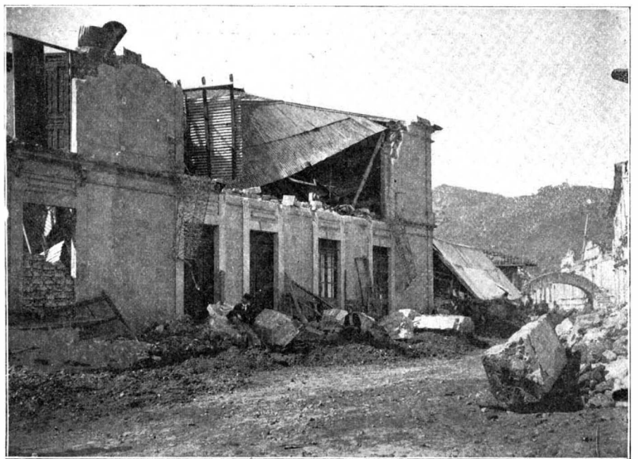
Remains of a House Belonging to a Wealthy Citizen, in Motazan Street.
