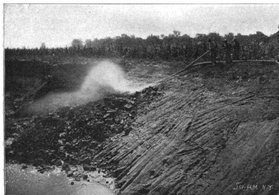
Hydraulic Grader at Work on the Bank.
