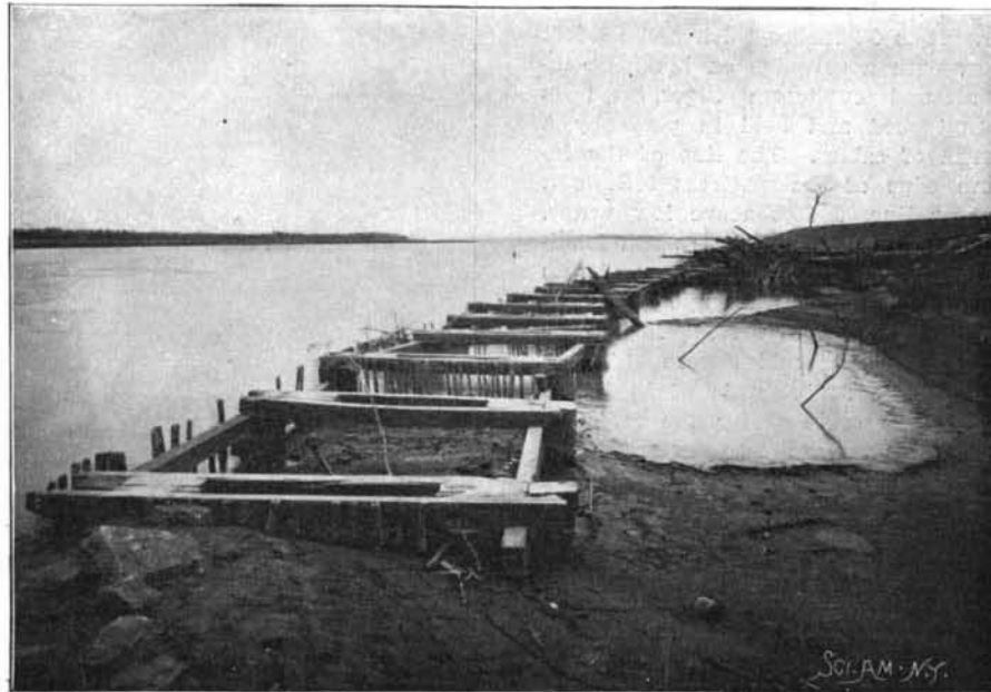
Government Dike to Prevent Scouring the Bank.
