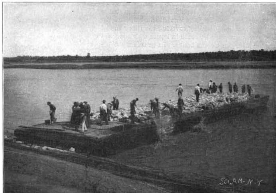
Sinking the Mat by Dumping Rock upon it.
