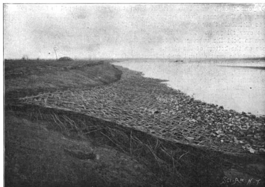
Eastern End of the Mat Completed and Sunk.
