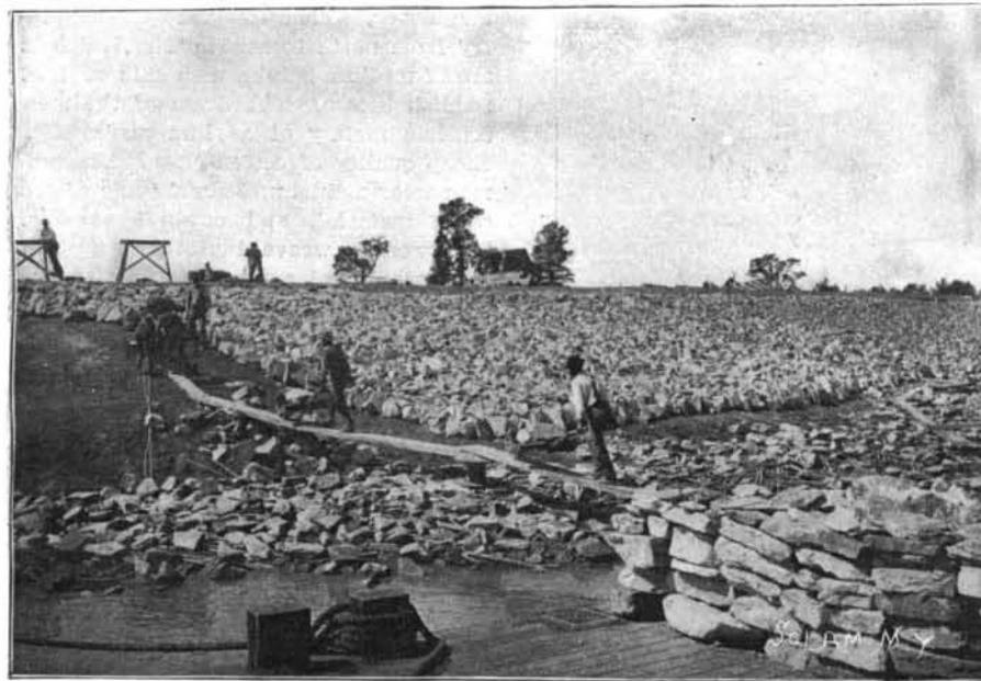
Paving the Bank.
