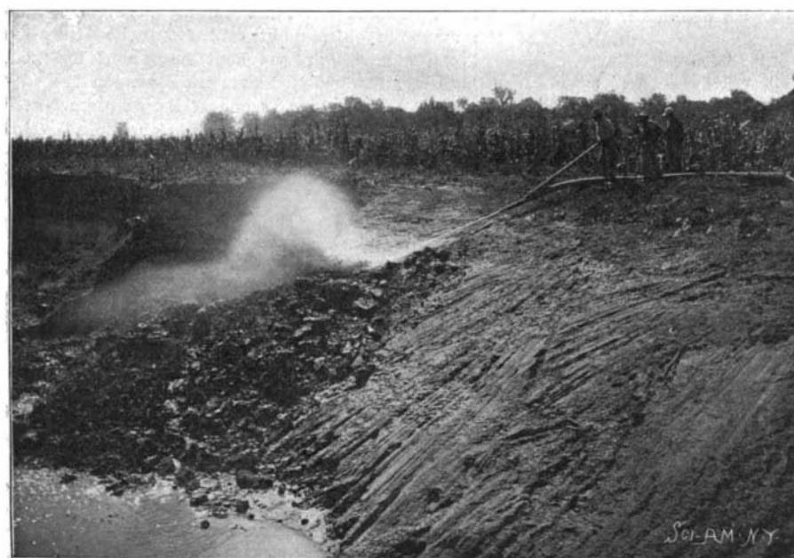
Hydraulic Grader at Work on the Bank.
