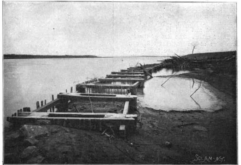
Government Dike to Prevent Scouring the Bank.
