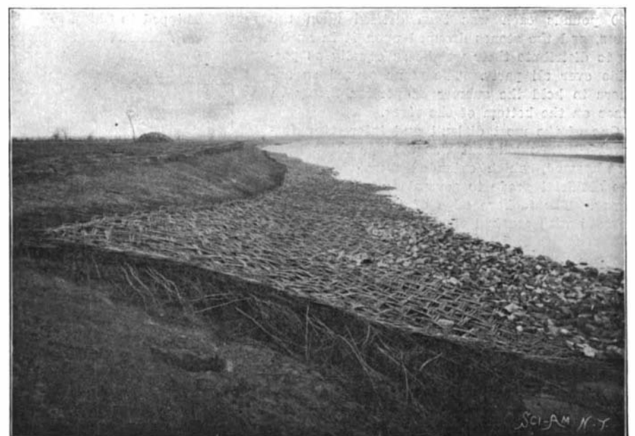
Eastern End of the Mat Completed and Sunk.
