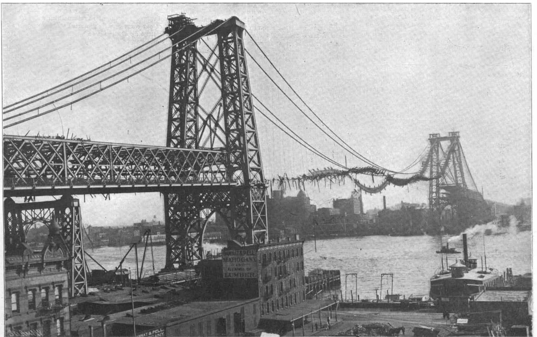
THE NEW EAST RIVER BRIDGE AFTER THE FIRE. THE MANHATTAN SIDE, WHERE FIRE OCCURRED IS IN THE FOREGROUND.—[See page 344.]
