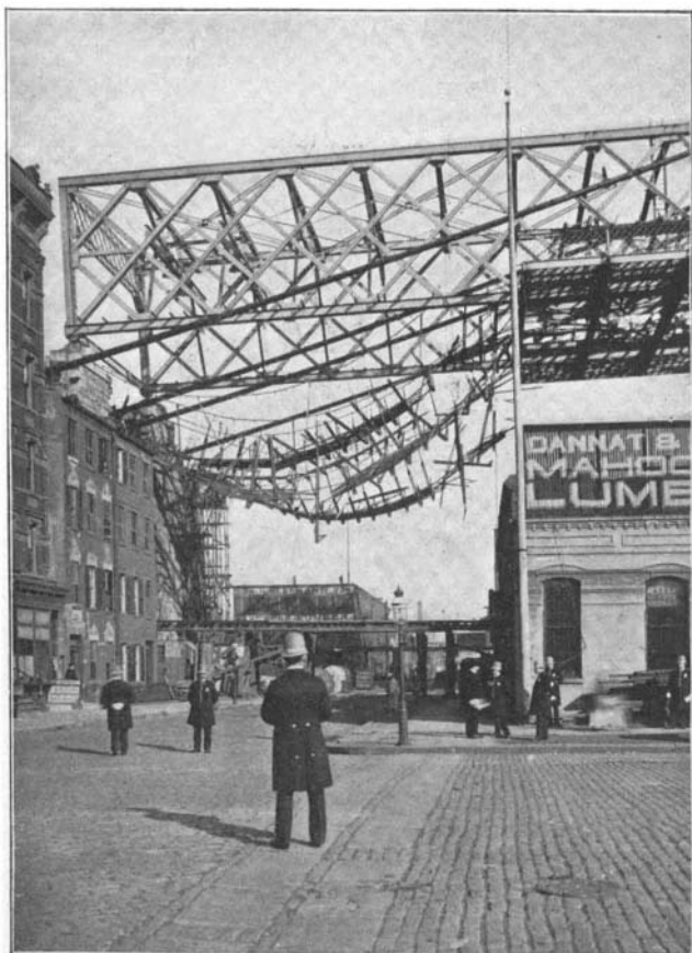
WRECKAGE OF FOOTBRIDGE AT MANHATTAN ANCHORAGE.
