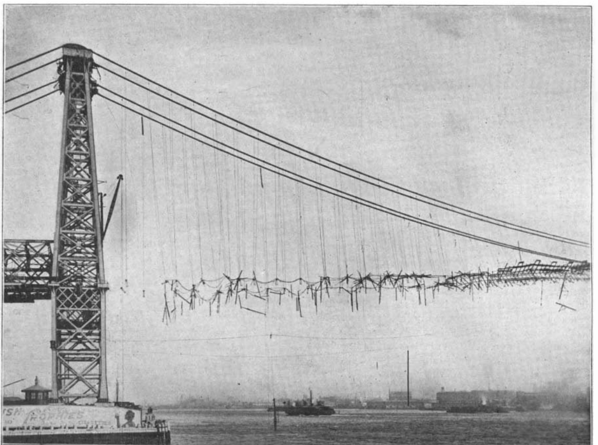
THE WESTERLY HALF OF MAIN SPAN, SHOWING WRECKAGE HELD IN THE SUSPENDER CABLES.
