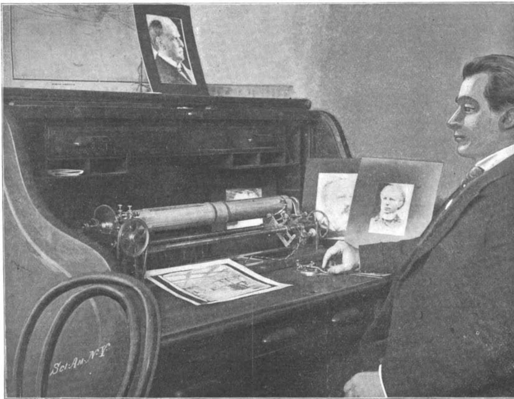
One of the Electrograph Machines, Showing Morse Key.
