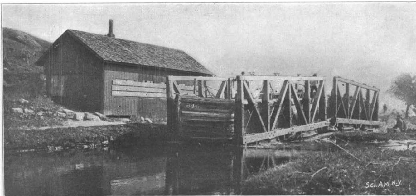
At the Summit of an Inclined Plane—Car and Boat Entering Upper Reach.
