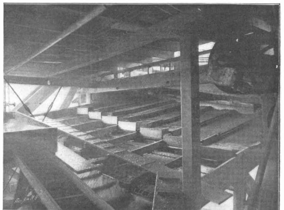
THE GOLD-SAVING TABLES OF A CALIFORNIA DREDGER.
