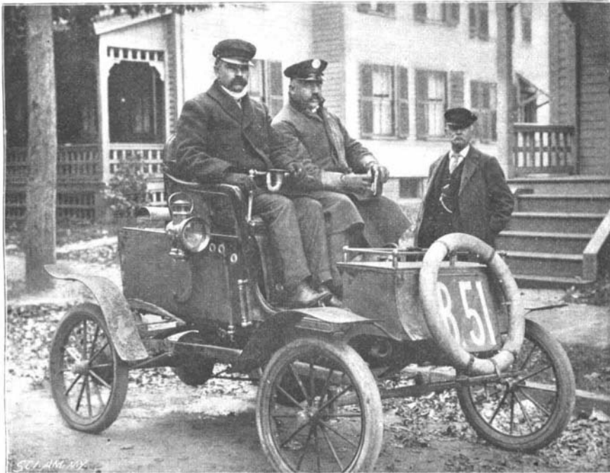
Stearns Steam Stanhope with Tubular Wheels.
