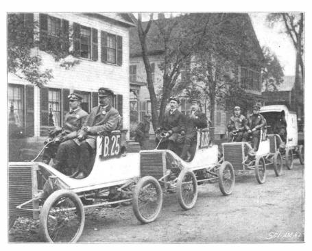
White Steam Stanhopes and Delivery Wagon, Showing Condensers Arranged in Front.
