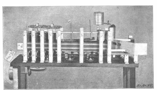
A MACHINE FOR SEALING ENVELOPES,
