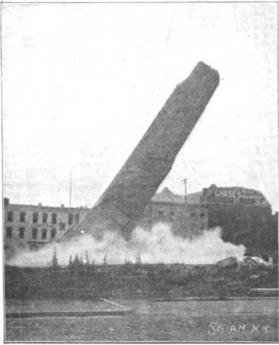
RAZING A BIG STACK WITH DYNAMITE AT WASHINGTON, D. C.
