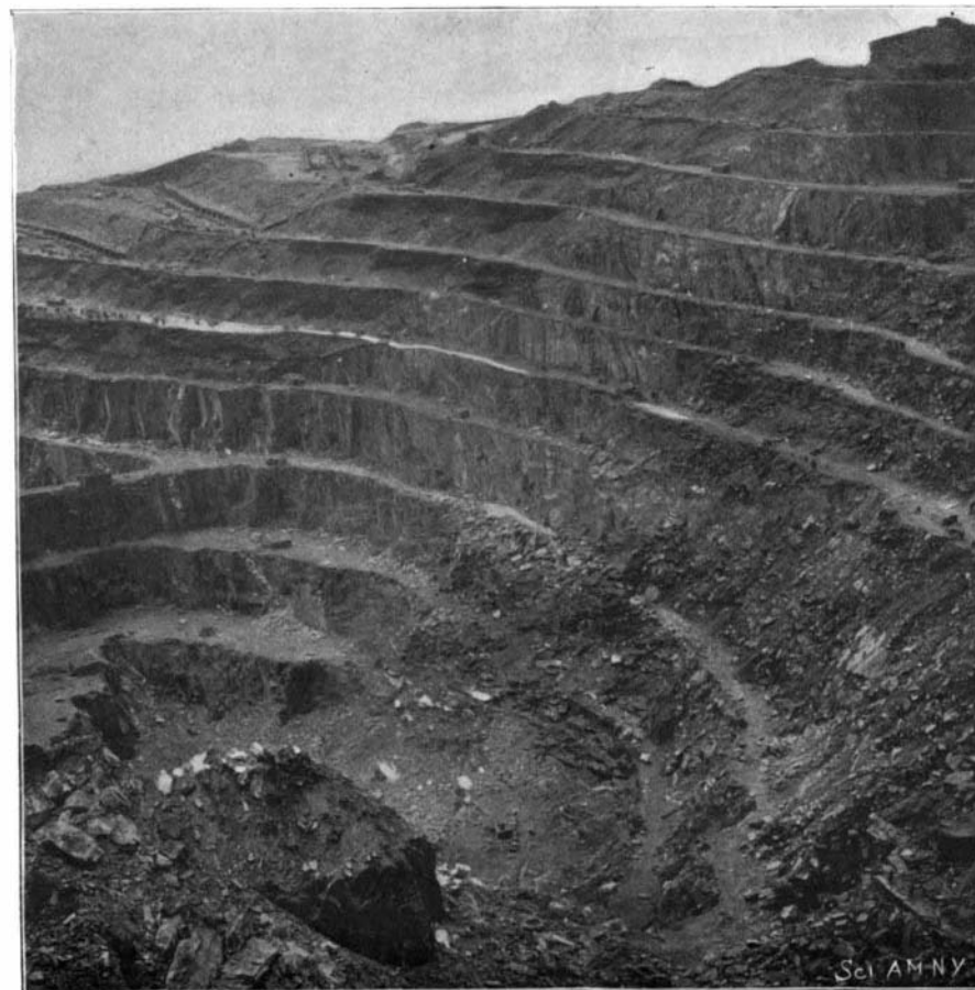
Fig. 2.—THE QUARRY AFTER THE PINNACLE WAS BLASTED AWAY.
