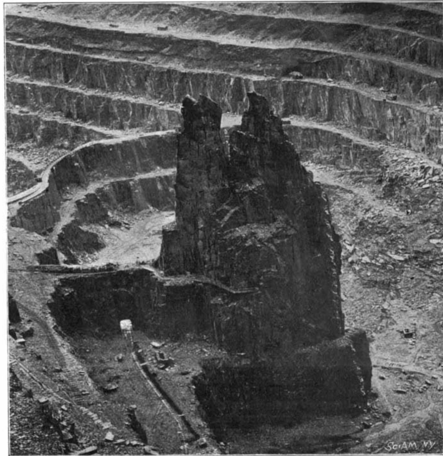
Fig. 1.—A 125,000-TON PINNACLE, 75 FEET HIGH, IN LORD PENRHYN'S SLATE QUARRY. BEFORE BLASTING.
