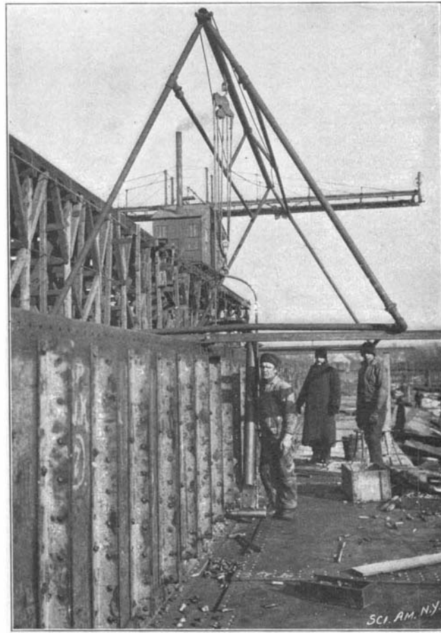
PNEUMATIC YOKE RIVETER, WORKING ON CENTER KEELSON.
