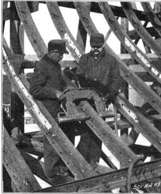
RIVETER AT WORK ON SIDE FRAMING.
