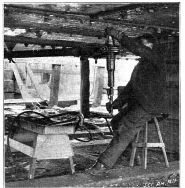
SHELL RIVETER WORKING ON THE BOTTOM.
