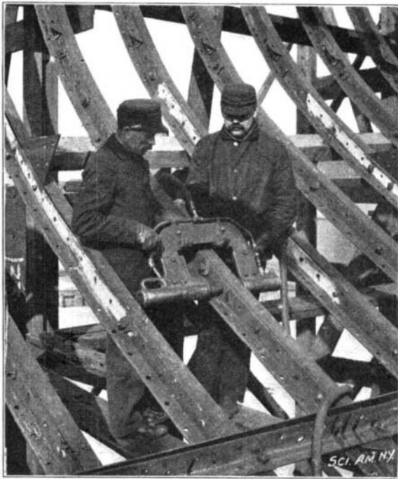
RIVETER AT WORK ON SIDE FRAMING.
