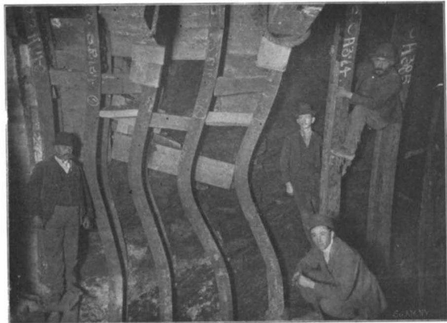
Heavy Steel I-Beams Yielding Under Pressure of Slacking Material.
