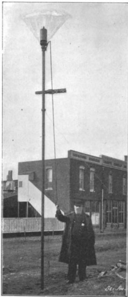
FIRE ALARM WHISTLE OPERATED BY NATURAL GAS.
