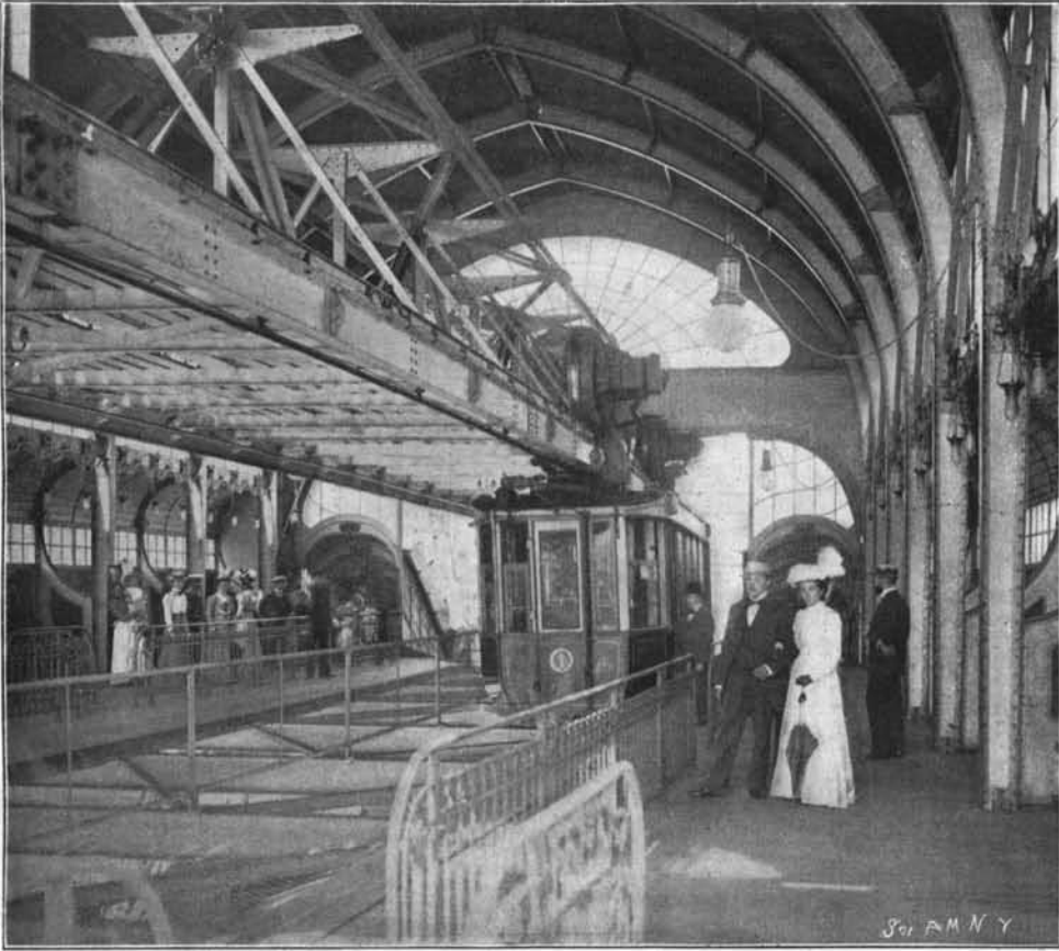
Interior of Doppersberg Station.
