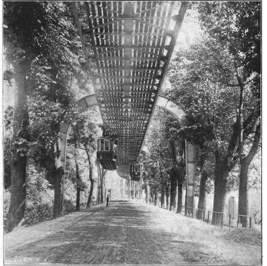
The Highway in Elberfeld Sonnborn, Showing the Inverted U-Frames.
