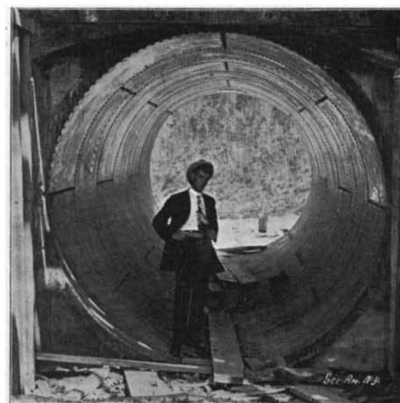
INSIDE PENSTOCK—9 FEET IN DIAMETER.
